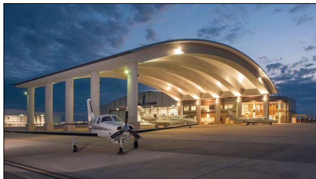
Houston Executive Airport's Jet Center. The airport, located in Brookshire, is currently adding a new hangar to its facilities. Internet photo.
