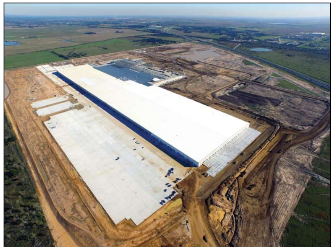
Aerial photo of the Daikin facility, currently under construction at Hwy. 290 and Kermier Rd., just east of Waller. Photo courtesy of Goodman Industries.
