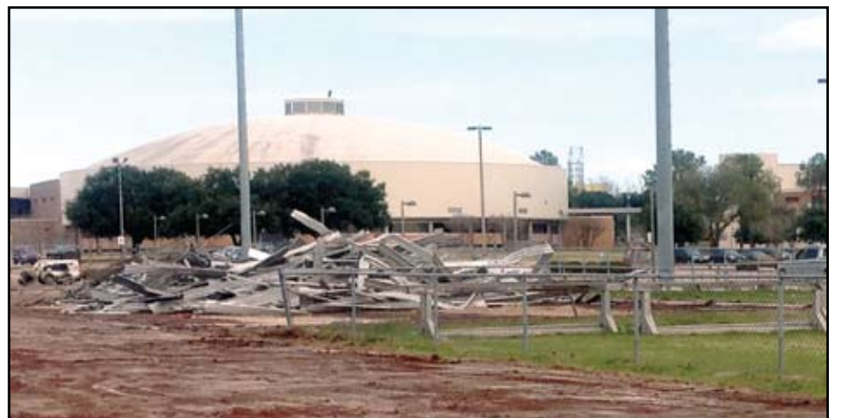
Demolition has begun of Blackshear Stadium at Prairie View A&M University. The old stadium will be replaced with a $53 million new state-of-the-art stadium and field house. Photo credit: Carrie Prazak-Gourley, The Waller Times.
